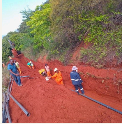
02 HILLSIDE PIPELINE TRENCHING
