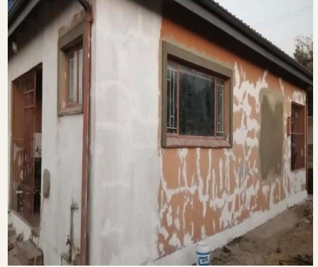
03 WALL & STRUCTURE REPAIRS
