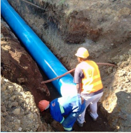
01 WATER MAIN PIPE LAYING
