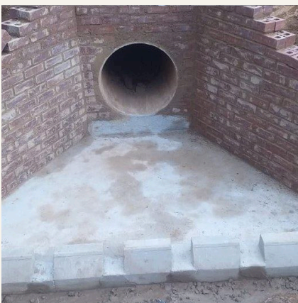
07 STORM WATER HEADWALL
