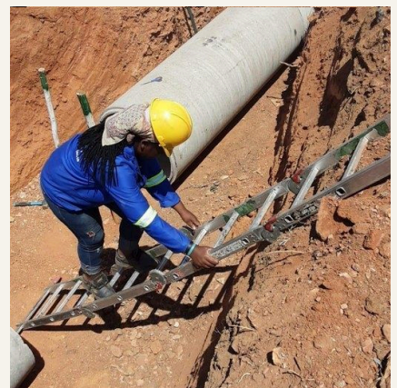
09 CONCRETE PIPE INSTALLATION
