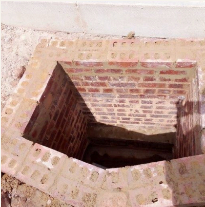
04 BRICK MANHOLE CHAMBER
